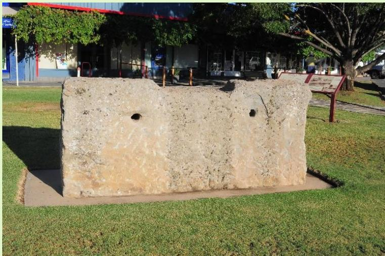
A portion of a Cornish pumping engine foundation stone for the cylinder of the engine. This stone is located in the main street of Burra. The two holes were for hold – down bolts.
