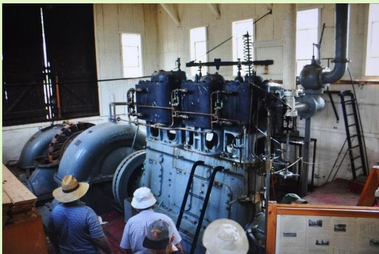
*Inside Millewa A pumping station. Triple expansion steam engine driving centrifugal pumps.*
